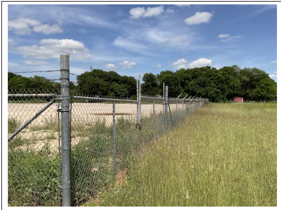
Photo 3 – View looking east along the southern edge of existing development.
